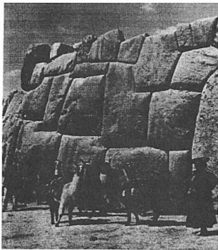
A portion of the wall at Sacsayhuaman.
